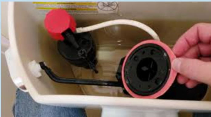
Example of someone replacing the flush valve seal.
